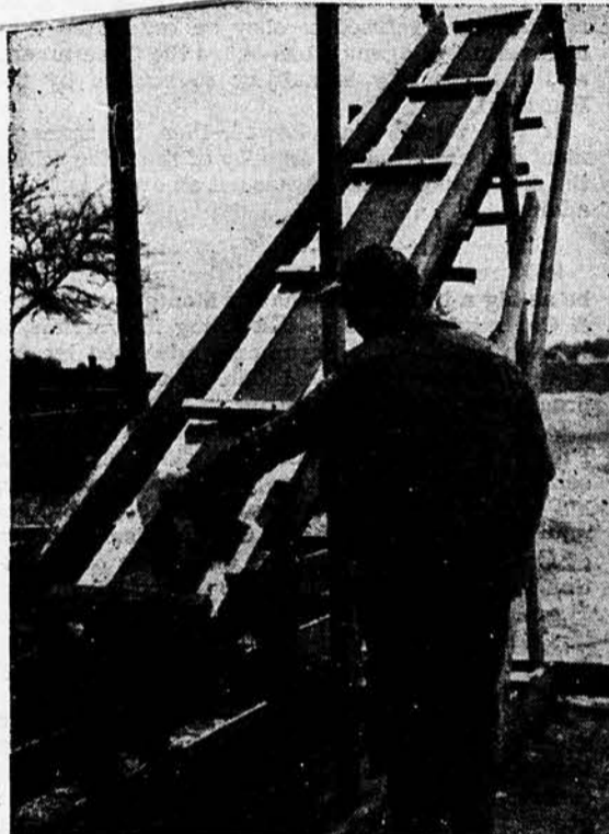
Homemade elevator for putting baled hay into the barn loft. The main working part is an old belt, with 2 by 2 wooden cleats attached.
