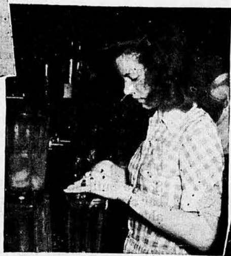
The Waring Blendor, being used here by Betty Anne Whitlatch, assistant chemist, looks like a malted-milk mixer and has much the same action. It removes some of the unwanted pigments from alfalfa extract.
