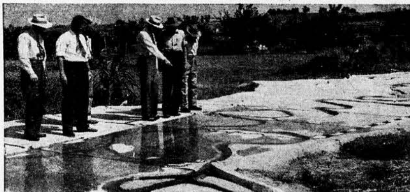
Army, state and college engineers watch the action of overflow results on the model under mild flood conditions. The picture shows how flood waters spread out over the valley.
