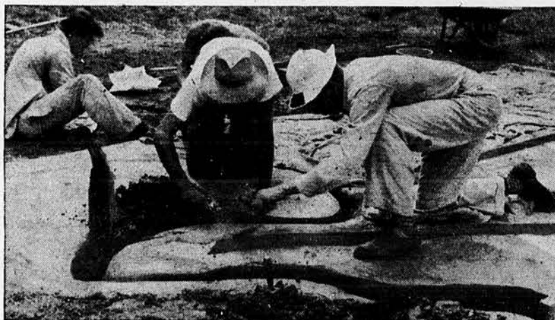
Engineering students here are shown constructing the model, which represents a valley 26 miles long and 2 to 3 miles wide. It is built on a scale of 8 feet to the mile.
