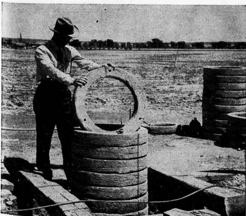
They may look like big "lifesaver" mints, but these structures are homemade segments for an irrigation well casing. Made by Sam Eitzen for his irrigation plant in Gray county, the concrete rings are shown at the well with Willis Wenrich, county agent.
