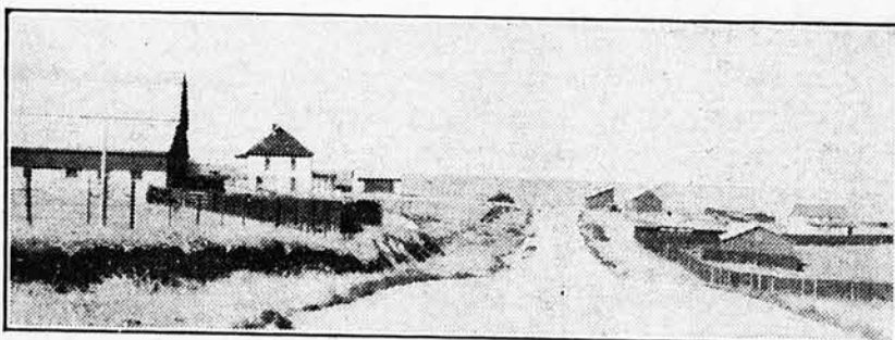
A good county highway now divides the ranch buildings of the J. T. Woods ranch in Logan county. At left is house and barn and beyond part of the thousands of acres of short grass. At right, sheds and corrals, flanked by meadows which provides winter hay.
