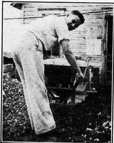
Manager Harold Hansen, of the Marion County Creamery, learns by doing. Assisting with the concrete work, to gain ability to direct later projects.
