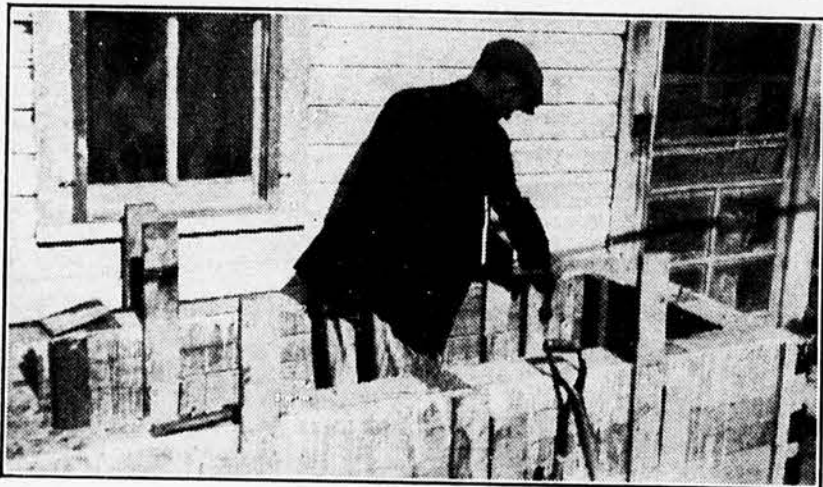
D. P. Kasper removing bolts which allow collapsing of forms without damage to them.
