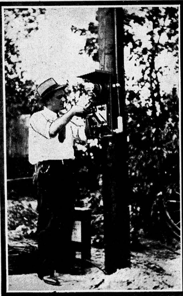
(Above)—Photo showing pole type entrance as center of electrical distribution system on farm of W. H. Zimmerman, Eudora, Kansas. This type of entrance is found quite convenient and satisfactory for farm electrification purposes.
