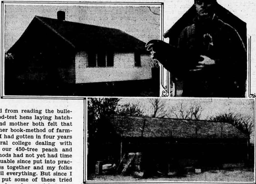
Highline Electricity Provides a Number of Electrical Conveniences in the Home That W. Clarence Fulton, Harper, Hopes to Finish This Spring. Right Top, You See Him Holding One of His Choice Rhode Island Red Roosters. Below Is the 200-Hen Laying House With the Glass Substitute Frames Raised Inside
