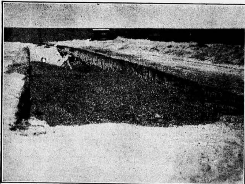
This photo shows a pit silo on the C. B. Campbell farm, near Lakin, 500 feet long, 16 feet wide and 10 feet deep, that was dug and filled at the same time. In other words the digging just kept ahead of the filling. Western Kansas does things on a big scale with present day power equipment
