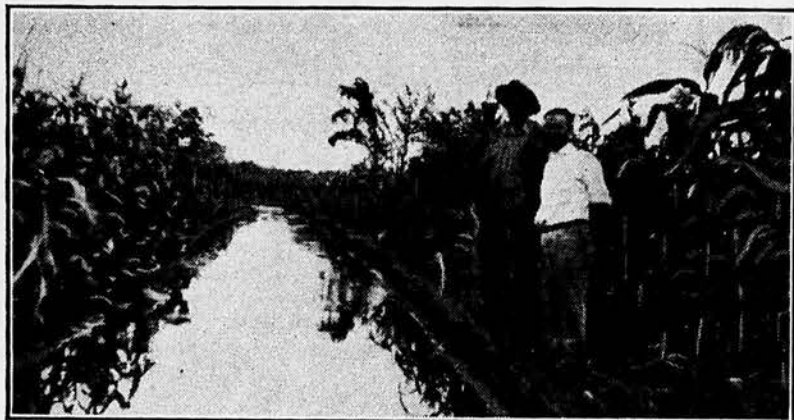
H. A. Ploughe, Jefferson County, Will Husk 75 Bushels of Corn to the Acre This Fall, and Here Is the Reason—He Irrigated. The Photo Shows the Main Ditch Thru the Field From Which Water Was Carried Down the Rows. The Pumping Plant Used Was Capable of Supplying 6,000 Gallons of Water an Hour
