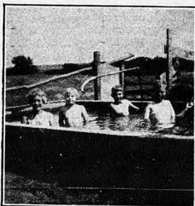
Farm Youngsters on the Hugh Holler Farm, McPherson County, Don't Worry About Hot Weather, Not Even When It Is 110 Degrees in the Shade, When They Are More Than Knee Deep in a Concrete Water Tank
