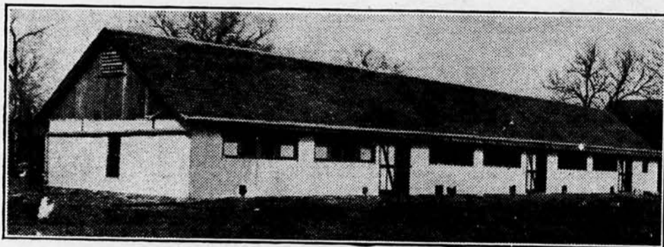
A 20 by 100 Foot Concrete-Board, Open-Front, Straw-Loft Poultry House on the H. S. Hiebert Farm, Near Hillsboro. One End Has a 10-Foot Feed Room. Under This Is a Concrete Cellar for Keeping Eggs Until They Are Sold. Equipment of This Kind Helps to Put Quality Poultry Products on the Market That Demand Top Prices
