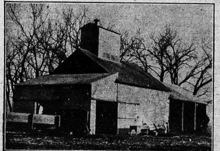
Proper Equipment Leads to More Profitable Farming by Virtue of Cutting Overhead. This Elevator on the W. A. Long Farm Near Fowler, Makes It Possible for Two Men to Handle the Job of Lamb Feeding Instead of the Seven Required Before It Was Built. In Addition It Saves Considerable Feed
