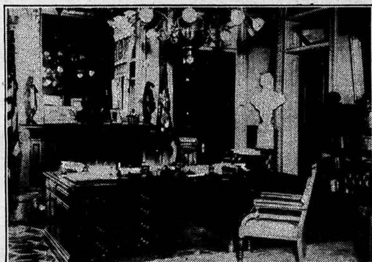
The Room Once Used as an Office by Gen. John J. Pershing in the State War and Navy Building, Washington, Which Will be Temporarily Occupied by President Hoover While His Office in the White House, Destroyed by Fire Christmas Eve, Is Being Rebuilt
