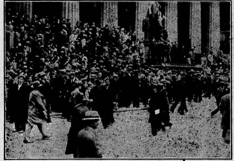
An Exciting Moment During the Recent Break in the Security Market in New York, When More Than 16 Million Shares Were Sold in a Day, a New All-Time Record. The Crowds Are Standing in Front of the Sub-Treasury, Which is Across the Street From the Exchange, at Broad and Wall Streets
