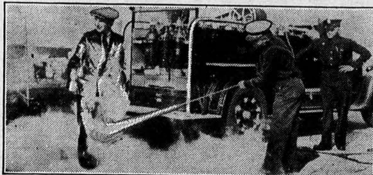
They Freeze Out the Fires in Los Angeles. Here's a Demonstration to Prove That the New Fire-Fighting Chemical, Carbon Dioxide Gas, is Not Harmful to Fabrics. The Gas Was Shot in a Freezing Stream Upon the Man's Clothing Without Damage to Man or His Suit
