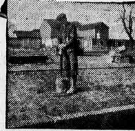
Tamping earth and rock fill prior to placing poultry house floor of concrete.
