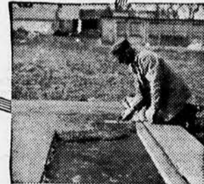
Placing layer of concrete over felt roofing paper. Paper eliminates dampness.
