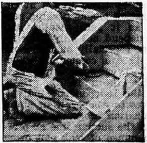
Note that beveled edge of form permits finishing top coat on step tread flush with riser of step.
