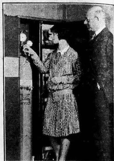
The New Oxyfier Which Will Keep One Man Alive for 220 Hours, or 10 Men for 22 Hours in Any Bank Vault. Chemicals Spread on Floor Absorb Carbon Dioxide Which is Exhaled
