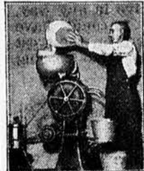
"Electric light for yards and farm buildings. Power for farm machinery and home electric appliances. All for only $1.25 a month." Robert McCue Mitchell, S.D.
