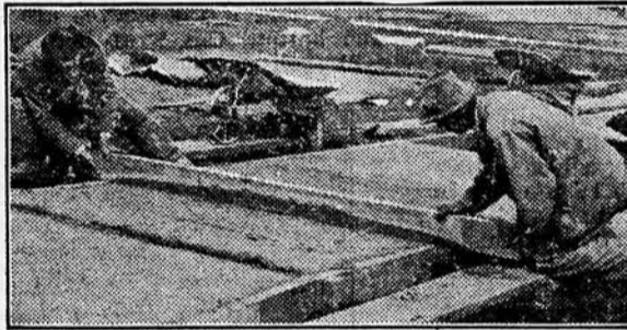
Leveling concrete with a board, known as a screed. The surface is then finished with a wood float, which provides a gritty, non-skid surface. The walk should be cured for a week. As soon as concrete sets, cover with straw and sprinkle with water.
