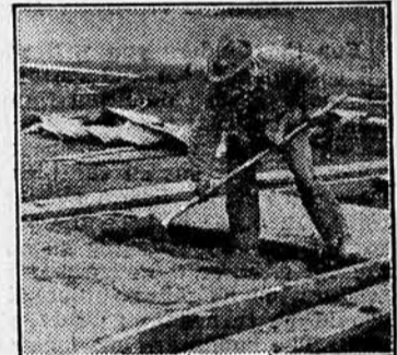
Use water sparingly in mixing concrete. Within reasonable limits, the less water used, the better the concrete.
