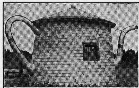
Here is a Building of Unusual Design, Being Used as a Filling Station. It is Made of Shingles, While the Spout and Handle Are Constructed of Clay and Plaster of Paris. The Spout Serves as a Chimney in the Winter
