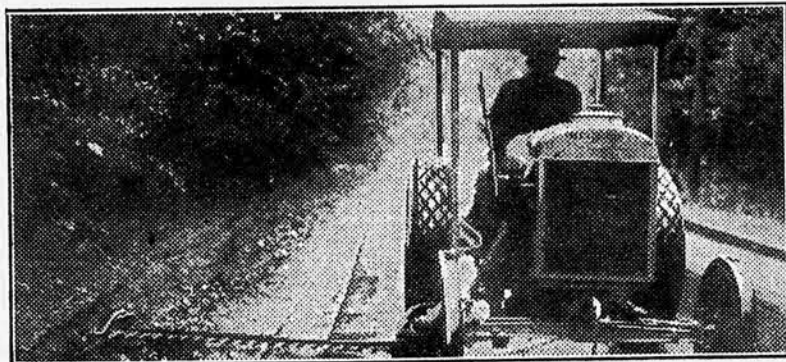
Photo Shows a Device Designed by the Highway Department of Multnomah County, Oregon, to Cut Weeds and Underbrush from the Sides of the Highway. It is Attached to a Tractor. The Speed is About Equal to That of a Rapidly-Walking Horse
