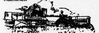
The McCormick-Deering Harvester-Thresher saves 20 cents per bushel over old methods in the harvesting of grain. It requires 15-30 power.
