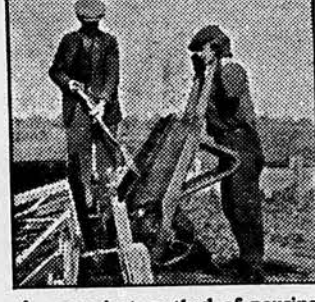
A convenient method of pouring concrete in the wall-forms. Note the movable boards to prevent wastage of concrete.
