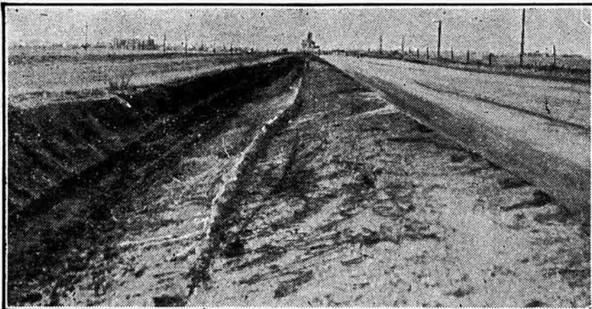
U. S. 40 North, East From Woodston, Where County Engineer Bodine Did Heavy Grading Work With His Two-Tractor System. The Road is Higher Than the Bordering Fields and the Wind Sweeps the Snow off Into the Wide Ditches
