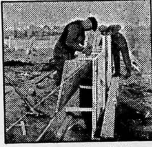
Forms for the wall are built over the foundation. Bolts to fasten the sill are placed in their proper position in the form.
