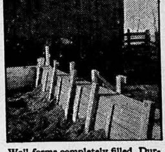
Wall-forms completely filled. During hot or cold weather, protection should be given the concrete while hardening.
