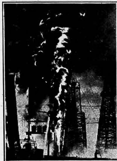
A Well in the Spindle Top Fields, Beaumont, Tex., Gushing Flaming Oil and Acrid Smoke. Damage Amounted to $100,000. The Fire Provided Plenty of Thrills and Hard Work
