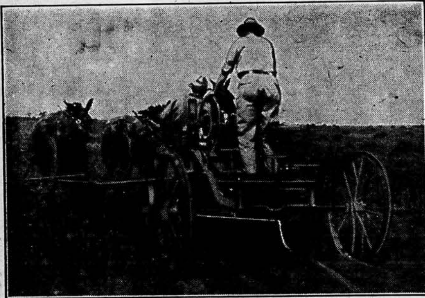
Walter Seematter, Marshall County, Driving. While C. K. Shedd of the Agricultural College Operates the Township Road Grader in Making Terraces to Prevent Soil Erosion on the Seematter Farm. The Grader Will Work in Most Cases, County Agent O'Connell Said
