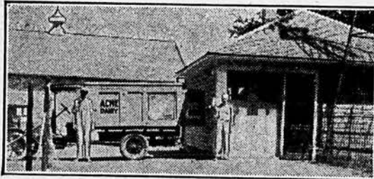
From the Dairy Barn the Milk is Rushed to the Milk House Where It is Cooled and Bottled. The Refrigerator Truck, at the Left, Makes One Delivery a Day
