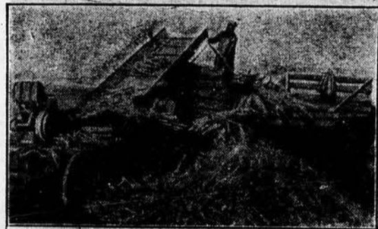
This is a Sorghum Tepper at Work on the Experiment Station Farm. It Cuts the Heads Off and Elevates Them to a Wagon Rack
