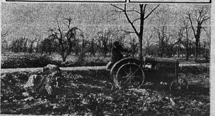
There are Many Practical Uses to Which a Tractor Can be Put on Farms in the Middle West During the Non-Rush Period, and Clearing Land is One of These
