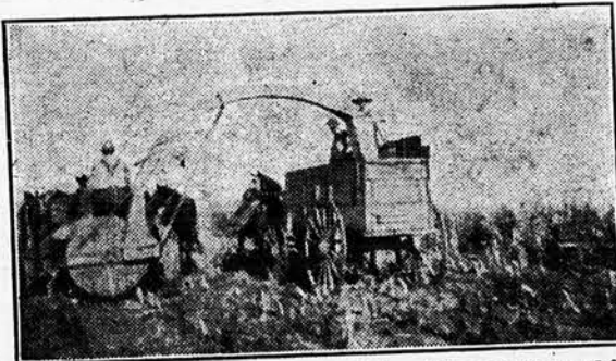
Three Men and Three Boys Make Silage With This Machine Which Cuts the Corn, Chops it Up and Delivers it into Wagon Boxes
