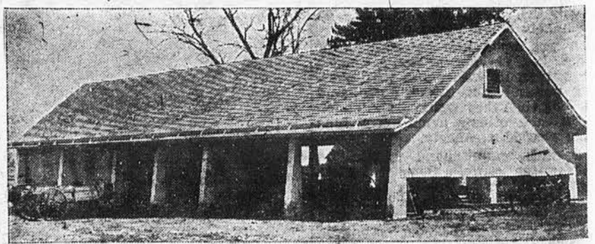
This Implement Shed Saved Its Cost in Five Years. When Farm Machinery Is Properly Housed, Depreciation on It is Greatly Reduced.
