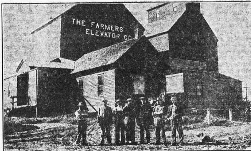
Co-operative Elevators Have Been Very Successful in Kansas, and They Have Done Much to Place Grain Production on a Better Basis.
