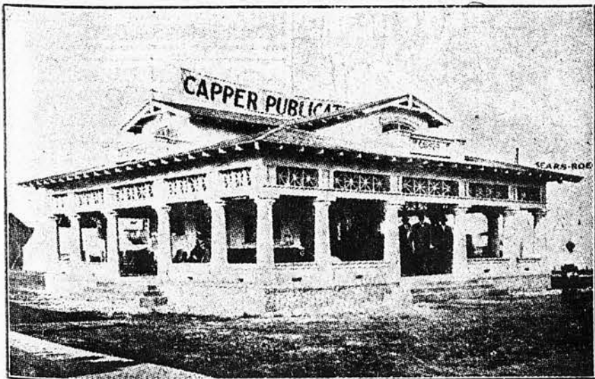
Home of the Capper Publications on the Kansas State Fair Grounds in Hutchinson Where Every Visitor Will Find a Cordial Welcome.
