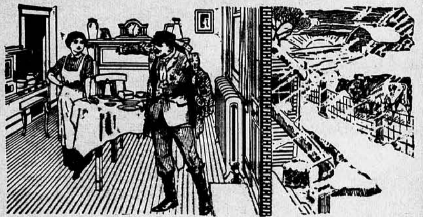
Cold, damp storms of early Spring never bother the cosy household warmed by AMERICAN Radiators and IDEAL Boilers, which furnish heat to suit the weather.
