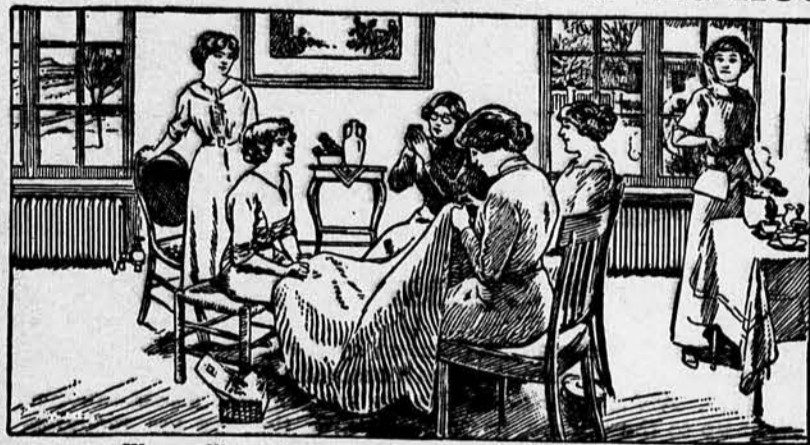
Women like radiator heating—it puts June in every room
