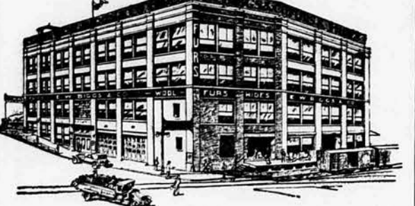
Our New Building Occupied Entirely by E. W. BIGGS & CO.
