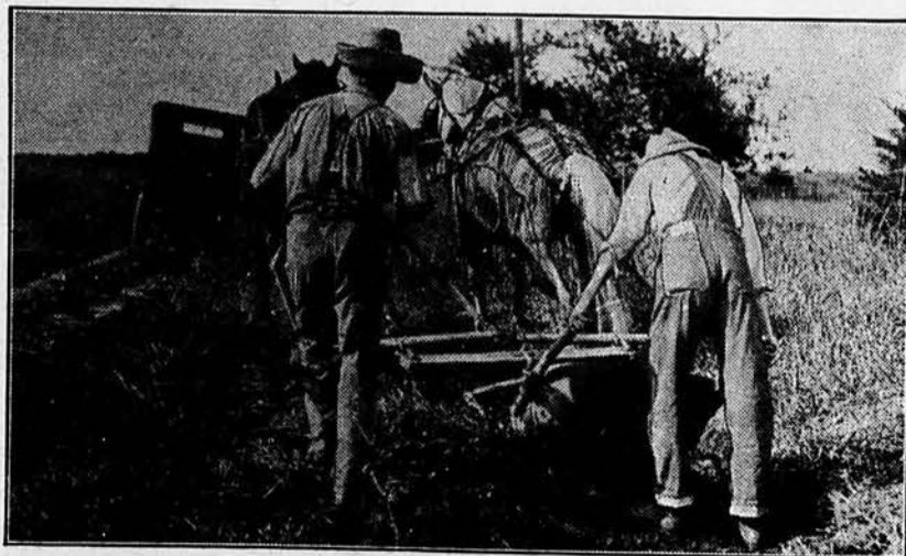
Frequent Repairs on the Roads Have Been Necessary to Keep Them Open For Hay Hauling, For the Rains Have Caused Many Washouts.
