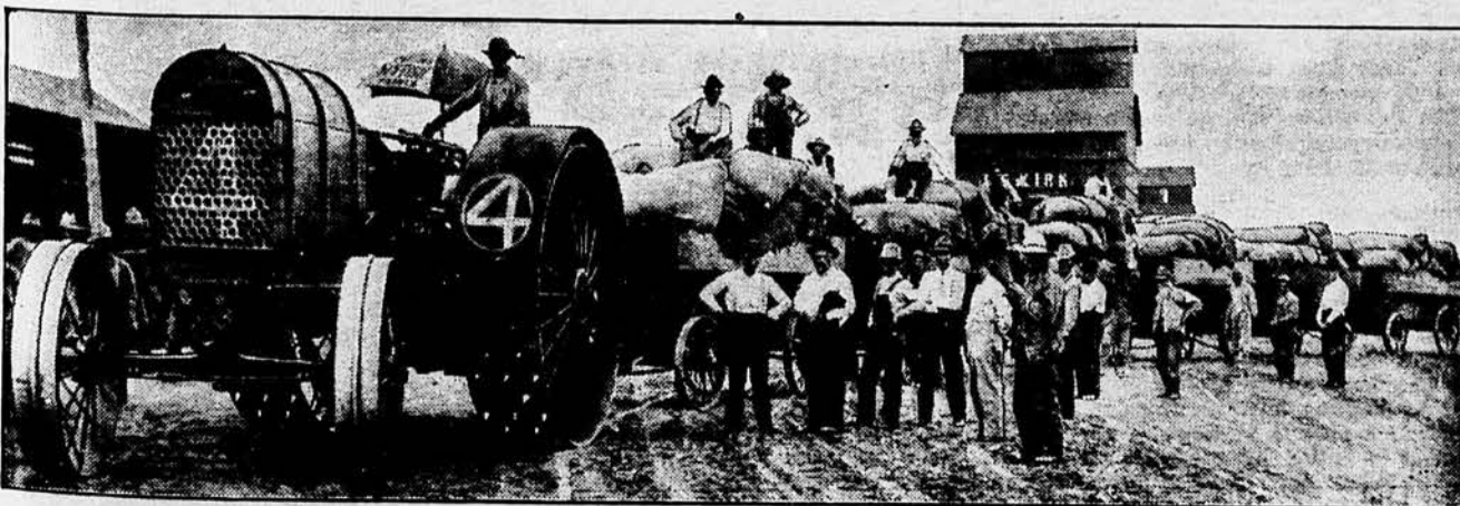
It Frequently Is Possible To Use Tractors Very Efficiently In Road Work. This Scene Is At Minneola, Kan.
