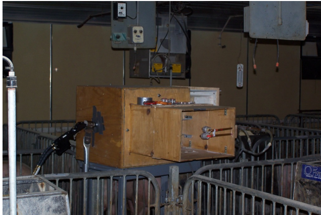
Figure 5. Photographs showing the scrubber inside the swine building during testing.
