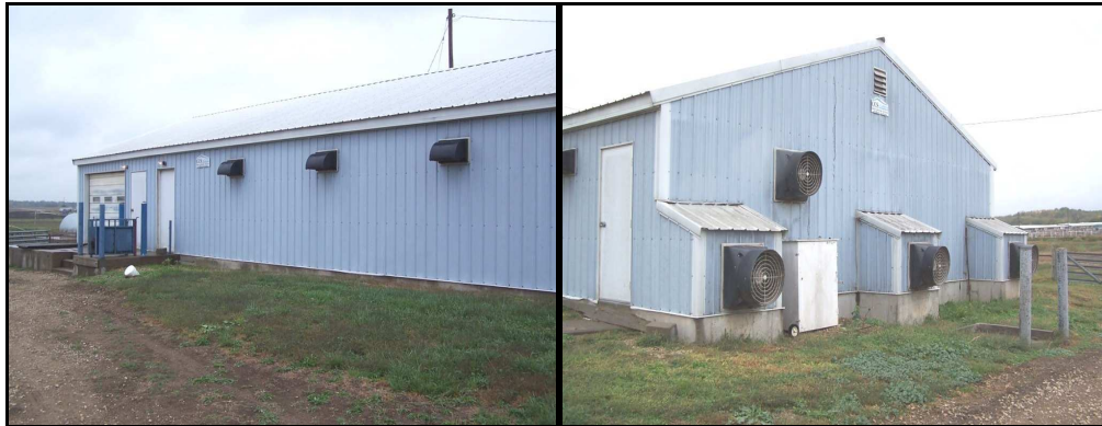
Figure 4-1 Exterior of the barn showing the air inlets and ventilation fans.
