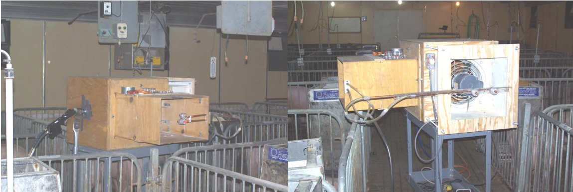
Figure 7-5 Photographs showing the scrubber inside the swine building during testing.
