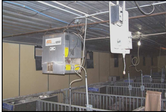
Figure 4-9 Supplemental heaters and environment control unit.
