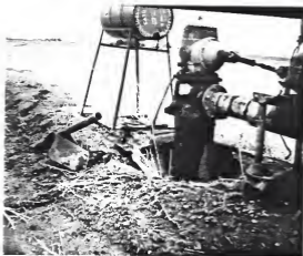
Figure 3. Protruding well casing in the Stewart area as a result of land subsidence
