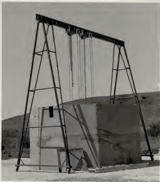
Plate 8. Completed source silo. A-frame crane is used for positioning of roof shields.
