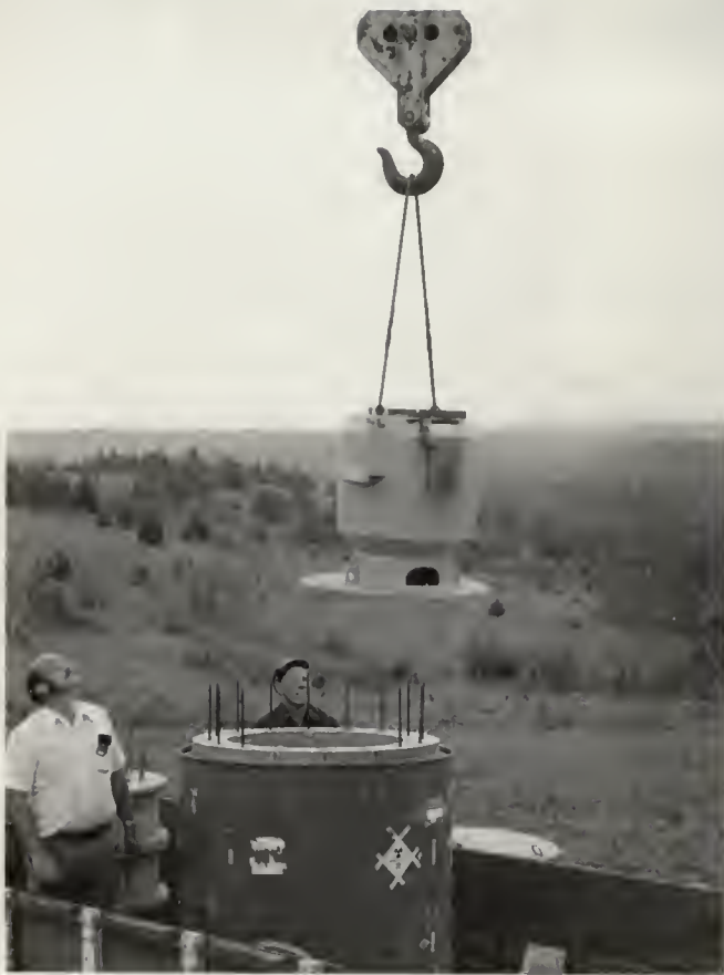
Plate 9. Source irradiator prior to placement in source silo.
