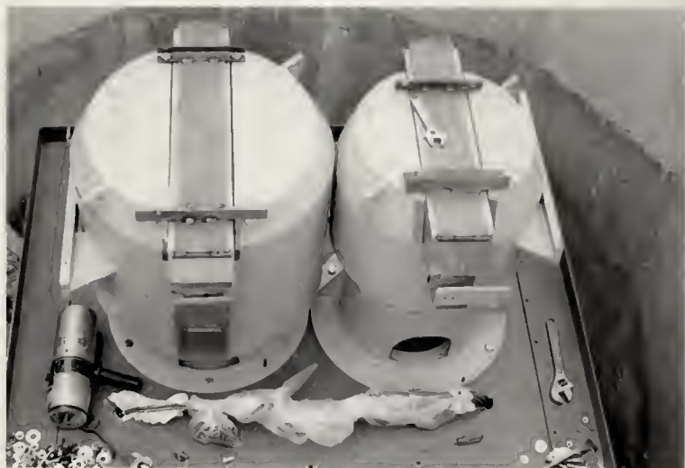
Plate 10. Source irradiators being installed on movable platform.
