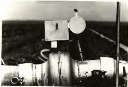
Figure 17. Three Way Slide Valve Mounted on a Flow Control Valve Located in the Field.
