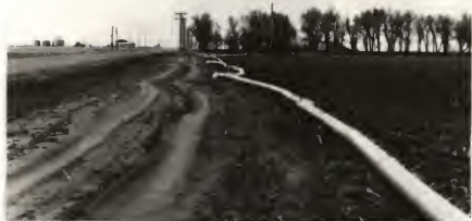
Figure 10. Gated Pipe Layed Out on the Upper End of the Field.
