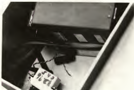
Figure 15. Inside of Flow Control Valve Box Showing the Servo and Ni-Cad Battery.
