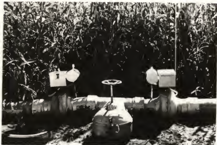
Figure 21. Hydrant and Flow Control Valves without a Solar Panel and Receiver Antenna Mounted on Flow Control Valve Box.
