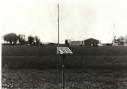
Figure 14. Solar Panel Mounted on a Bracket Supported by a Pole 8 Feet above Ground.
