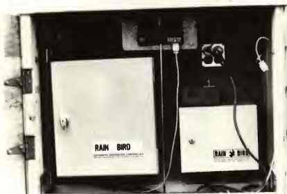
Figure 8. Inside View of Plywood Box Showing the Controllers, Transmitters, Power Supply and Electrical Outlet.
