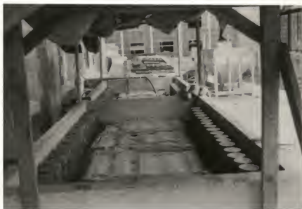
Fig. 17. View of bed after completion of molding one series of specimens. Moist burlap covered the beams and cylinders during the curing period.
