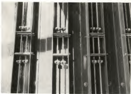
Fig. 16. Detail of beam mold ends. Note bond increasers and method of securing plate bulkheads.
