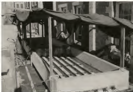
Fig. 18. The cured specimens were carefully identified before removal from the bed. Tarpaulin canopy kept bed and molds from becoming excessively warm during molding operations and early curing stages.
