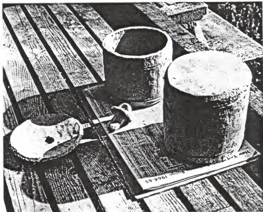
FIGURE 13: EXAMPLES OF SAGGARS USED BY JAPANESE POTTERS FOR THEIR RAKU WARE.
