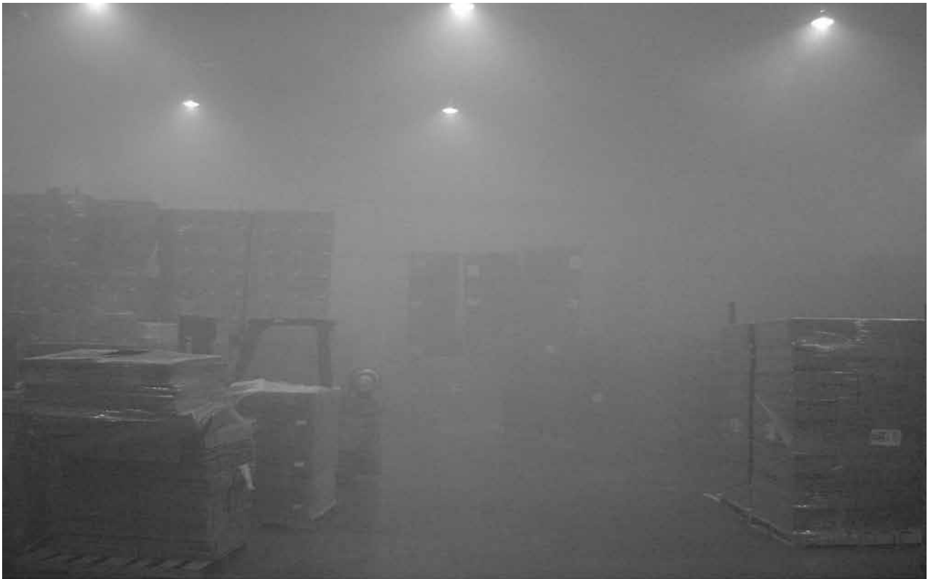
Figure 3. Dispersion of pyrethrin aerosol inside a food storage facility. The aerosol was dispensed from an application system installed in the ceiling, and the insecticide was dispensed outward from the nozzles. (Photo courtesy of F. H. Arthur, USDA-ARS-CGAHR.)
