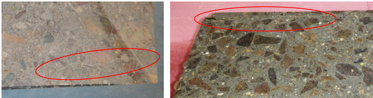
Figure 7.11 Cracking due to stress release from saw-cutting
