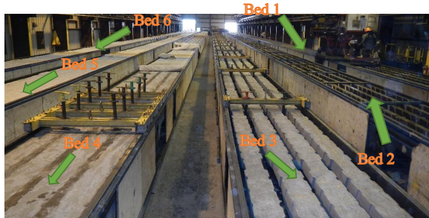
Figure 3.3 Casting beds in Plant B
