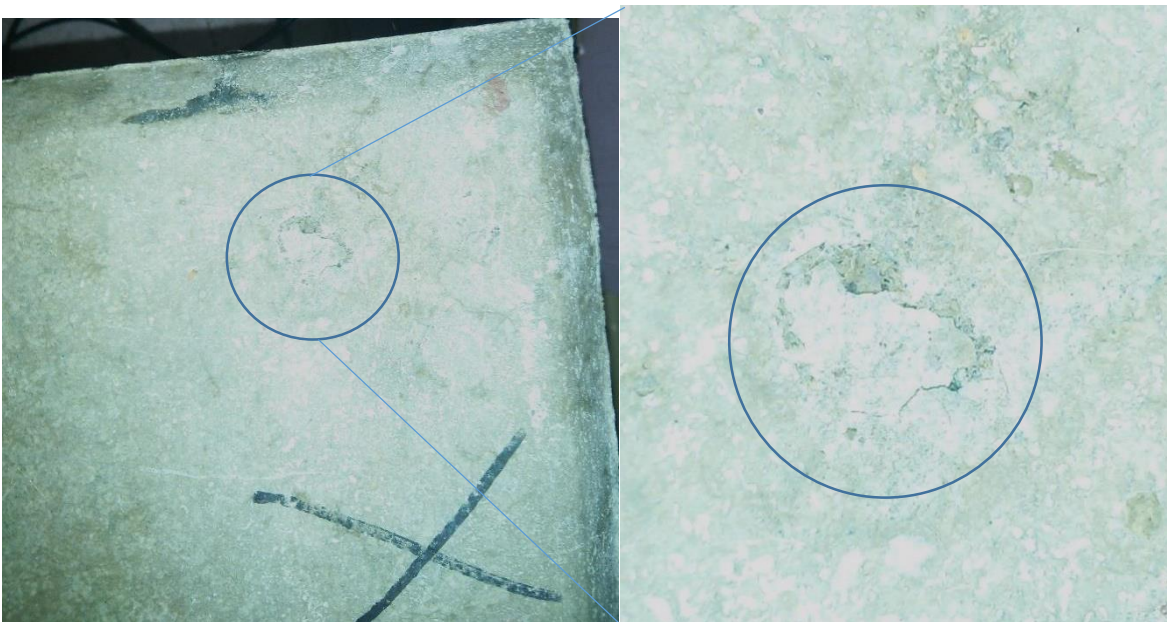
Figure 4.26 Small pop-out/crack in Tie #1-4397-F
