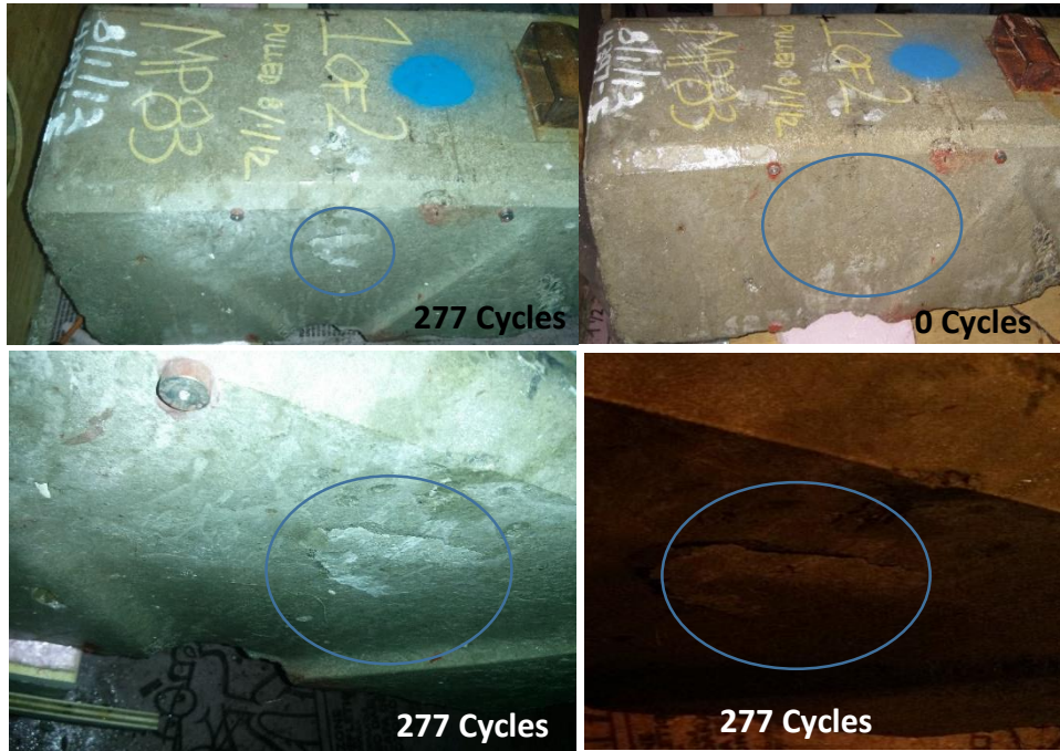
Figure 4.25 Tie #1-4397-F shallow cracking
