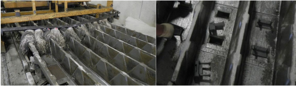
Figure 3.1 a) Forms cleaning and oiling, and b) shoulder installation in Plant A
