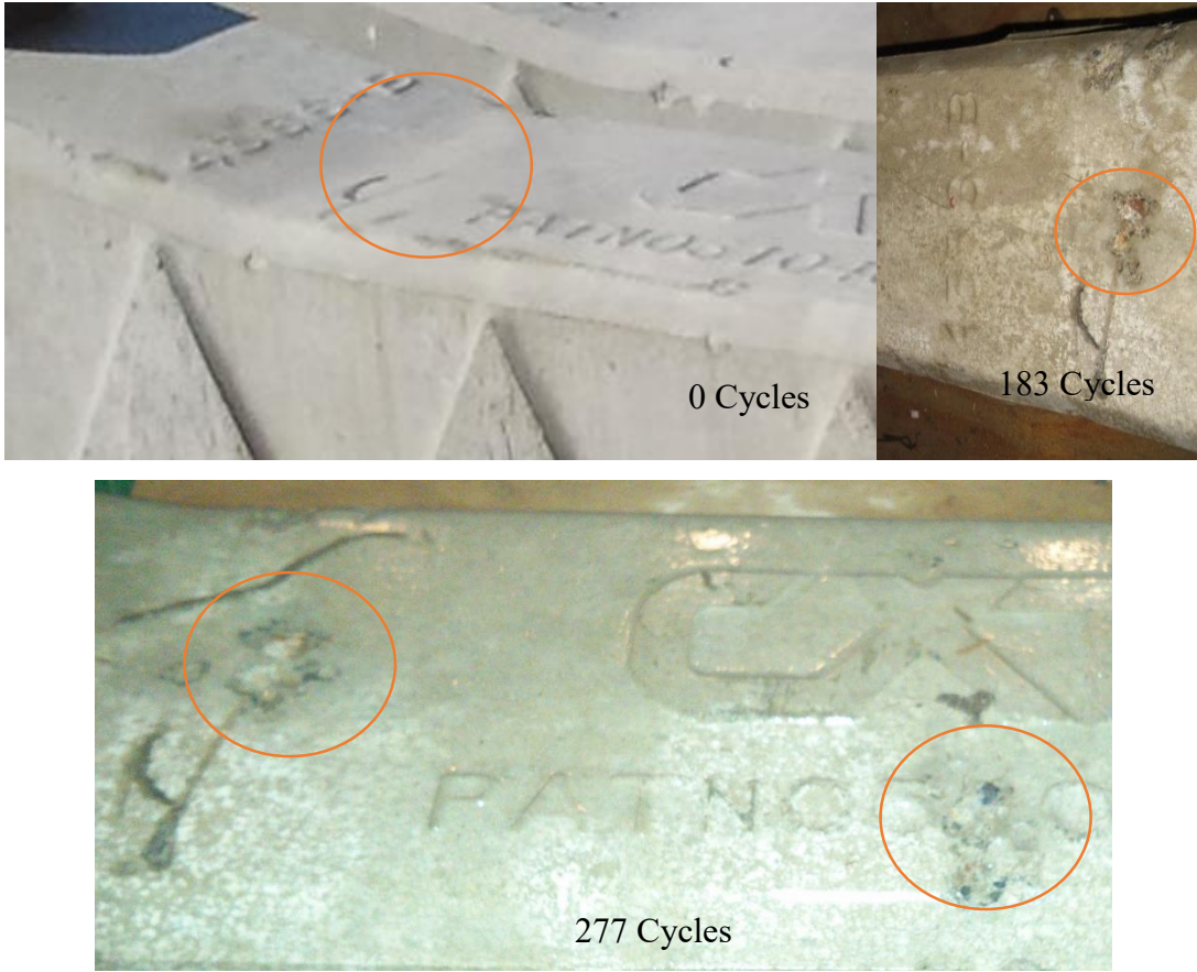
Figure 4.23 Tie #2-4386-B pop-outs and surface scaling
