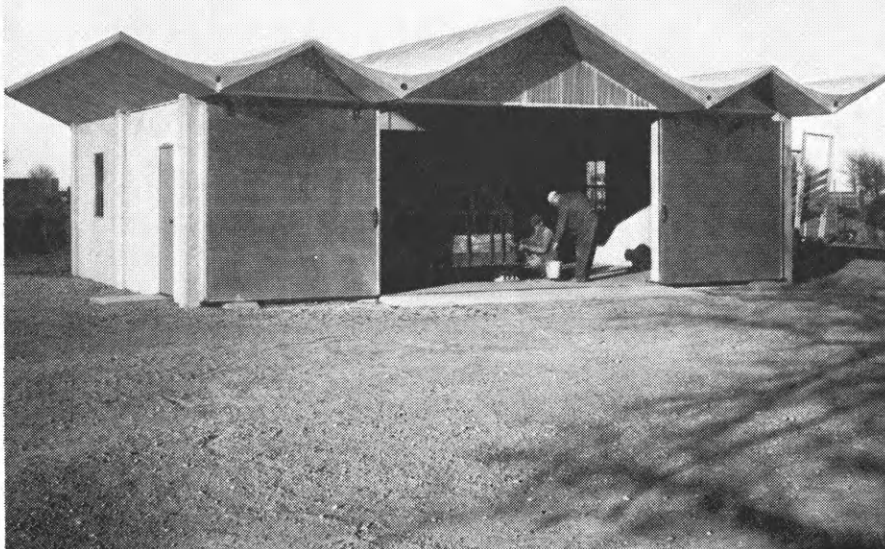
This all-concrete machine shed was such a success, the owner built four more buildings like it.
