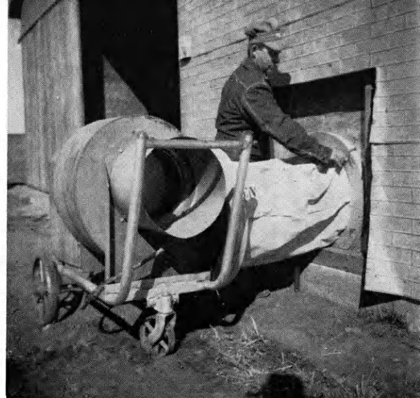
Low initial cost of equipment, low operating cost, and easy utilization are why this farmer is using forced natural air for grain drying.
