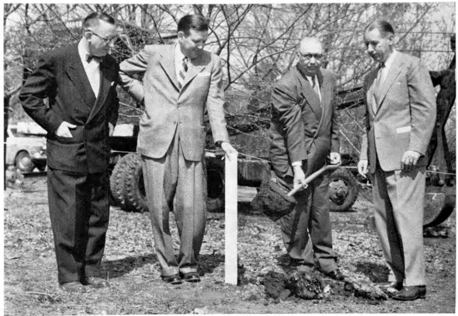
THE FIRST SPADE of soil for the new feed technology building is being turned by John Vanier, member of the feed milling advisory committee. Looking on from left to right are: Loren V. Burns, Pres. James A. McCain, and Dr. J. A. Shellenberger.
