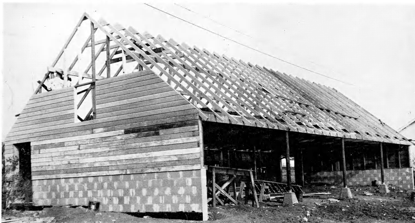
THE NEW BEEF SHED will probably be capped off with shingles by the time this picture is published. Bill Parker, the Ag Education major in charge, said they hoped to finish the 26x56 foot structure very shortly.
