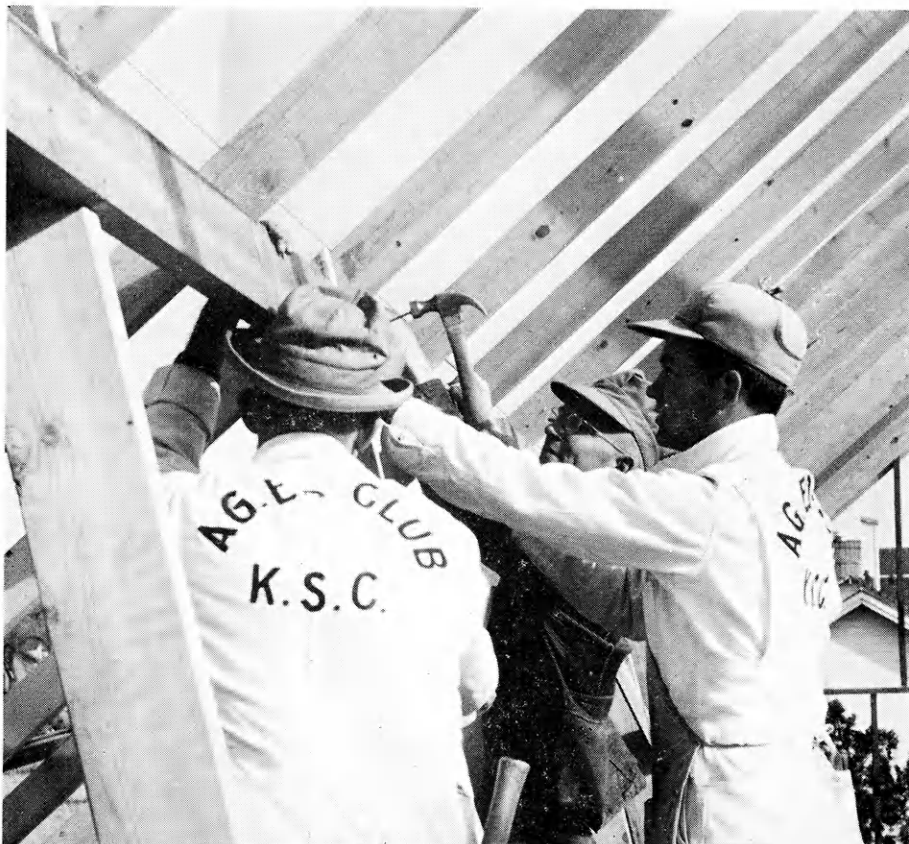
ENOUGH THUMBS for that hammer to hit something that squeals—that's the way the new loafing shed northeast of the beef barn has gone up. About 50 members of the Farm Buildings Construction class have put the shed up as a class project, using salvaged lumber for most of it. That's Harold Gentry with his back to the camera. Marvin Smith swings at the nail while Clarence Swallow assists on the far side.
